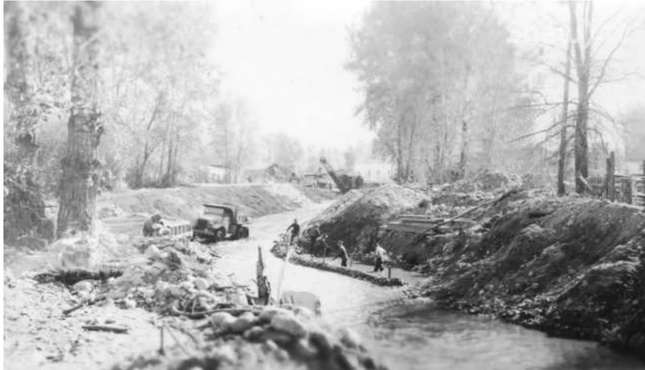
Construction of the channel lining (date unknown)
