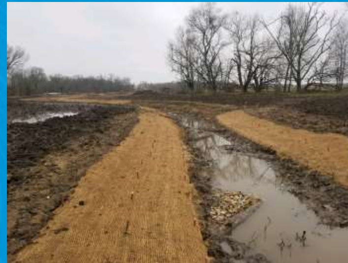
Log Constructed Riffle
