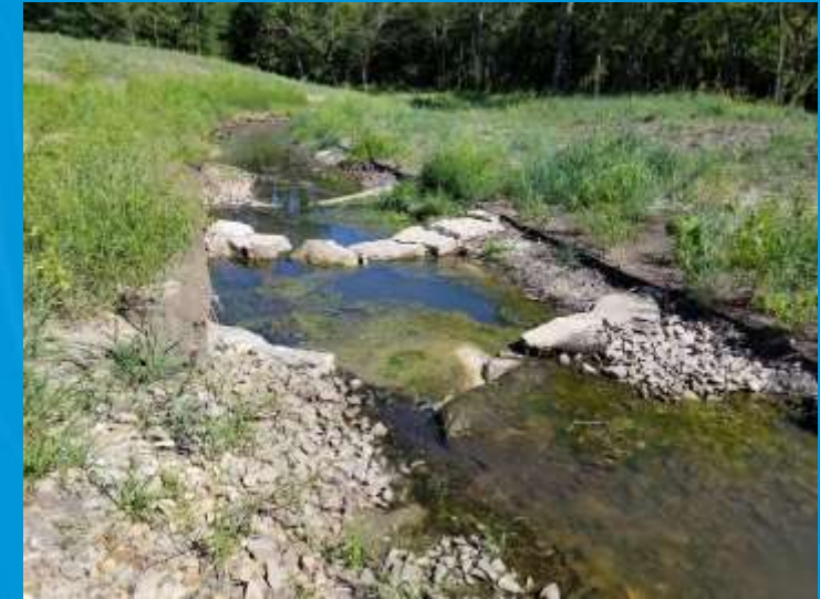
Boulder Constructed Riffle
