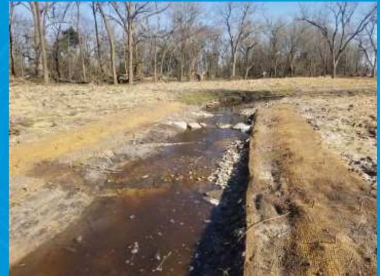
Log/Boulder Constructed Riffle
