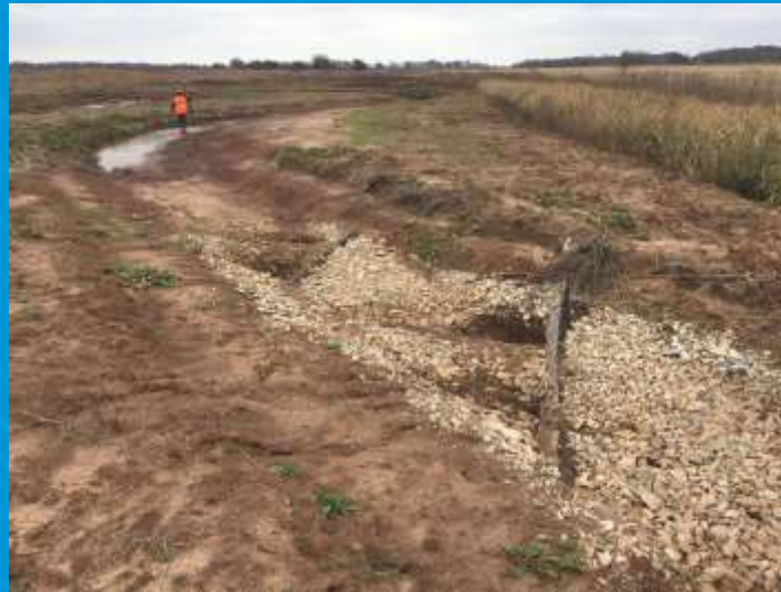
Log Constructed Riffle
