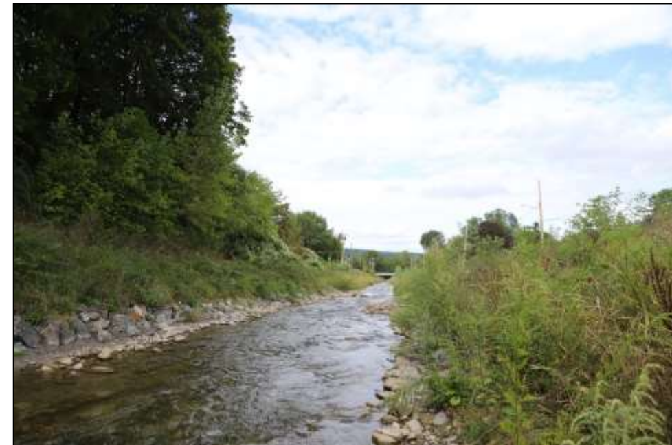
Top Right: Steele Creek, Ilion, NY, during construction, 2020 Bottom Right: after construction, 2022
