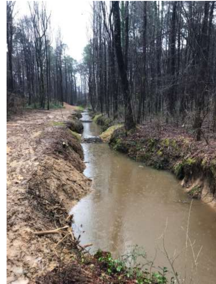
Construction Completed January, 2019
