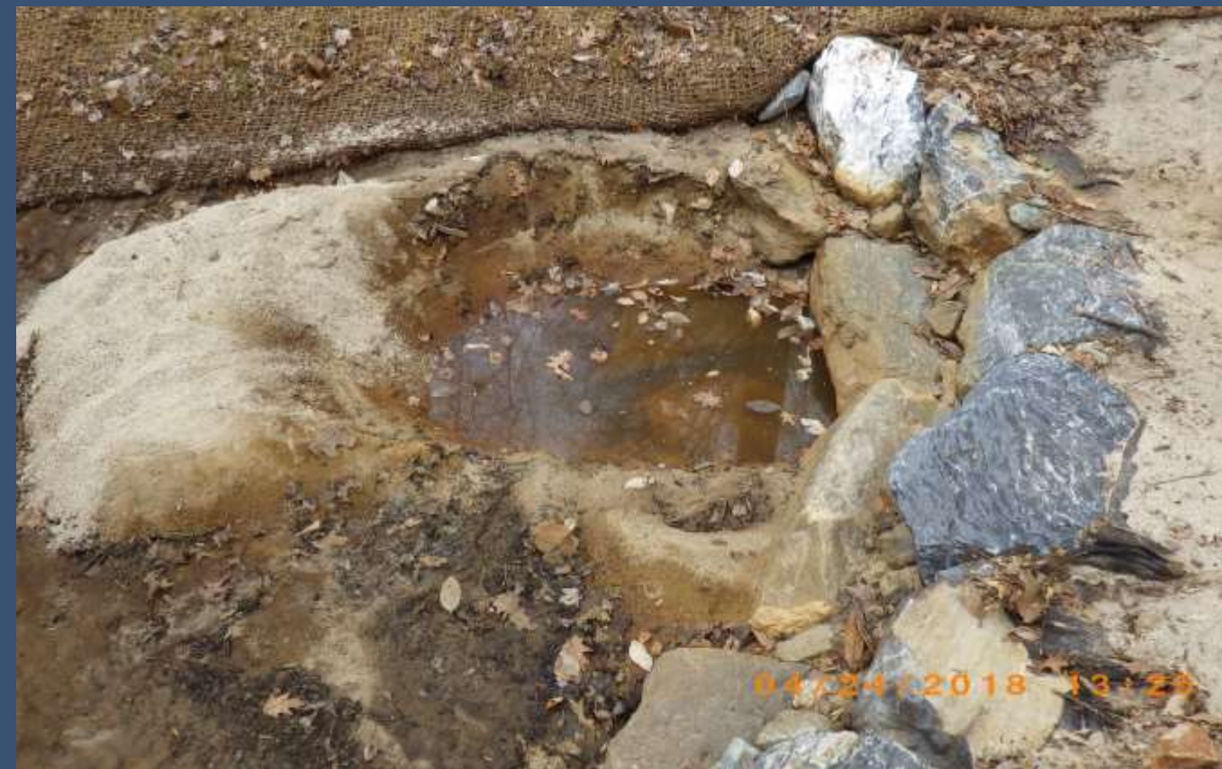
No Splash Rock = Sand Blow Out
