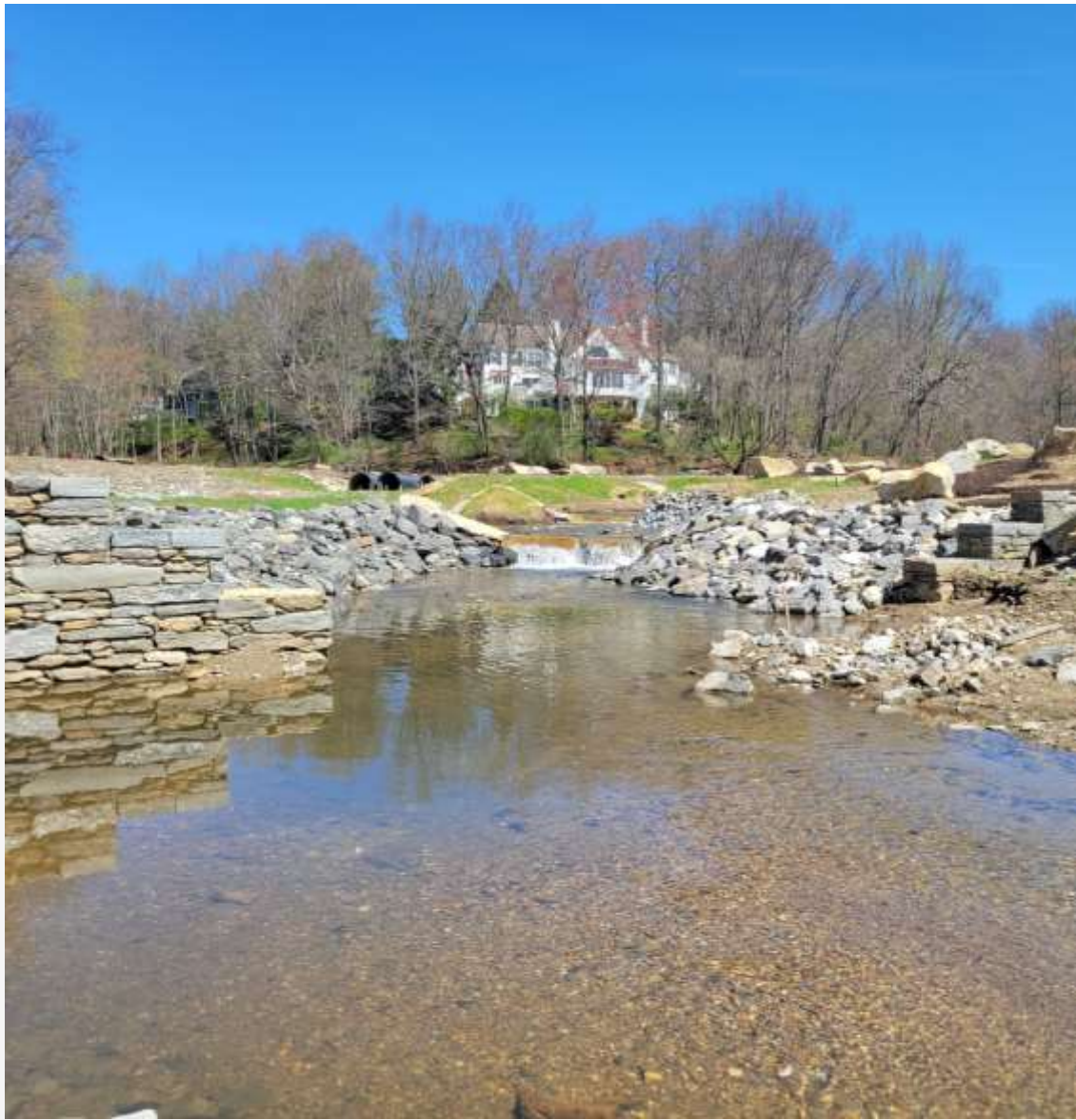
Aesthetic Stone Wall & Waterfalls
