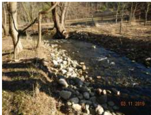
Constructed Riffles
