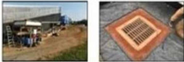
Test Setup and Installation (20% around 20" x 20" in size)
