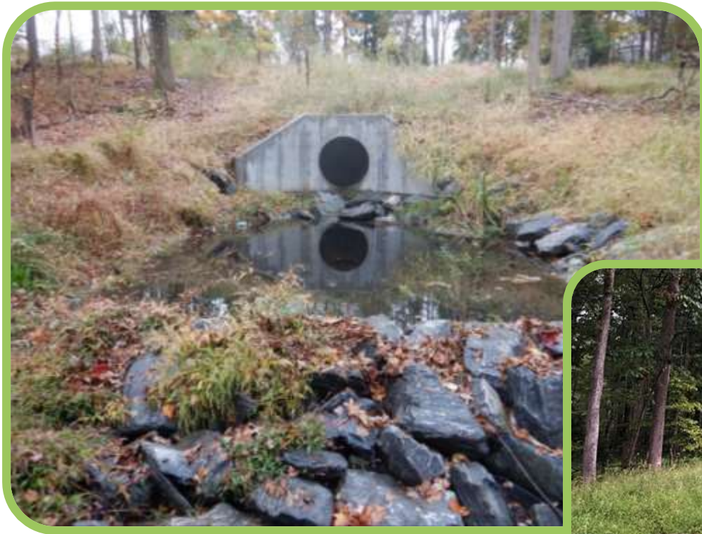
Left: Chasm resultant of failed level spreader structure. Above & Right: Photos of the restored SW infrastructure and repaired slope.
