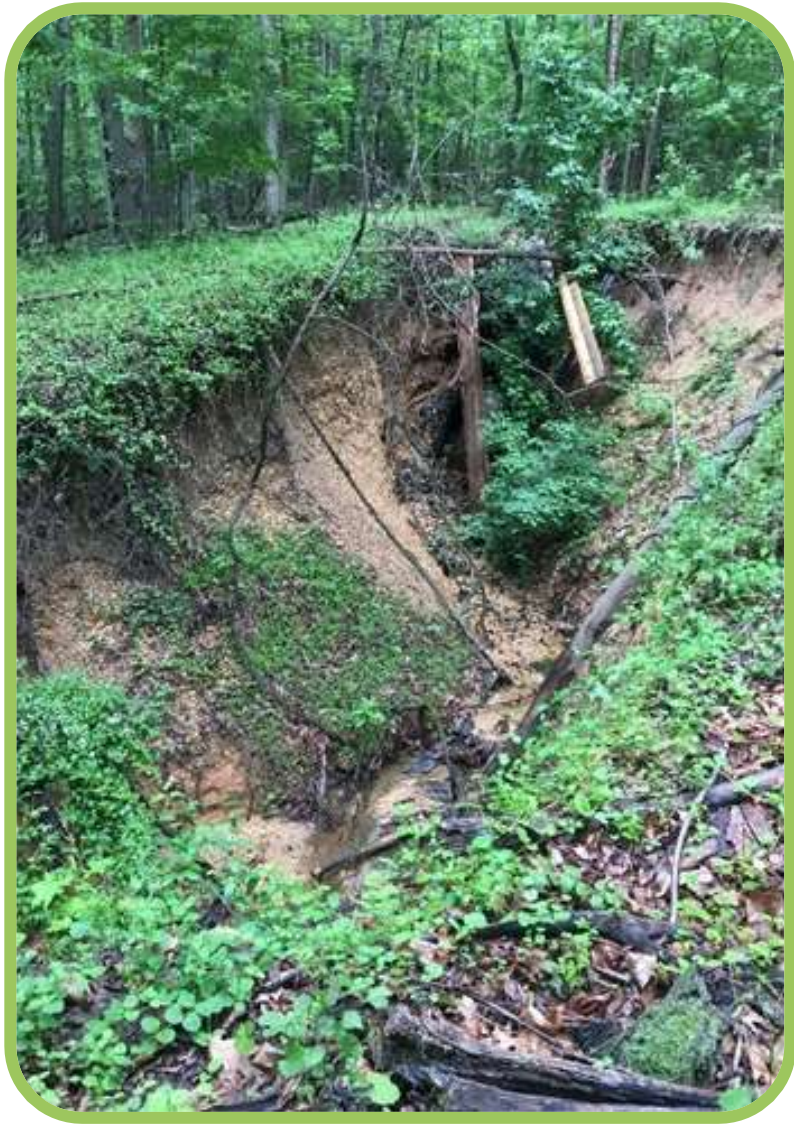
Left: Chasm resultant of failed level spreader structure. Above & Right: Photos of the restored SW infrastructure and repaired slope.
