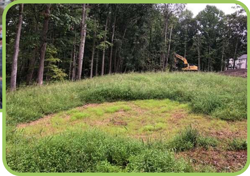
Left: Chasm resultant of failed level spreader structure. Above & Right: Photos of the restored SW infrastructure and repaired slope.
