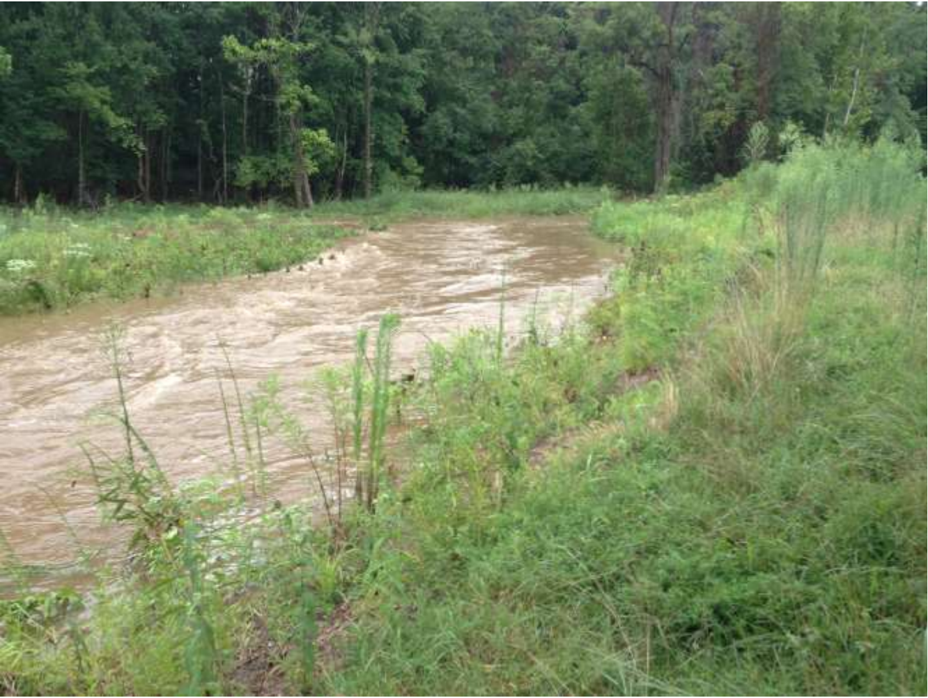
Outer Bend Erosion
