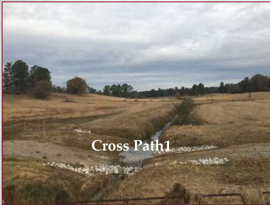
No fenced stream NRCS 381 - Stream Crossing
