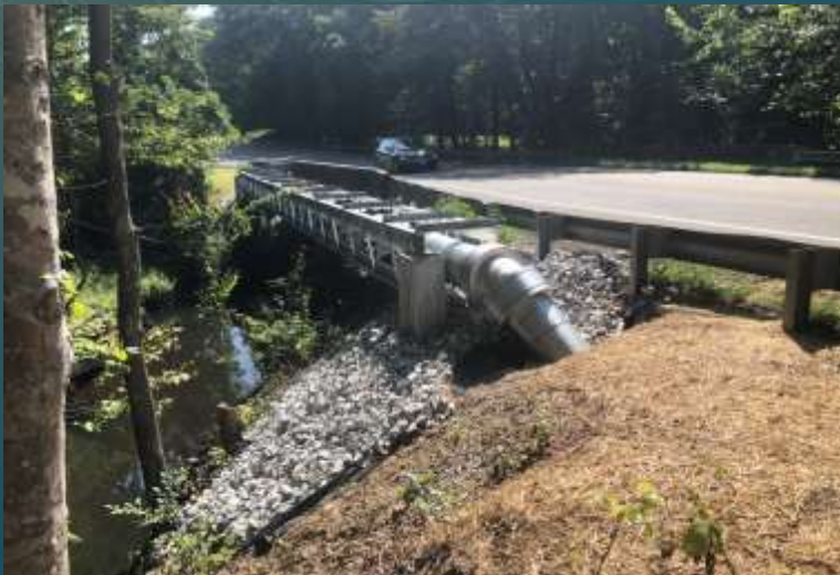
Emergency Water Line Repair
