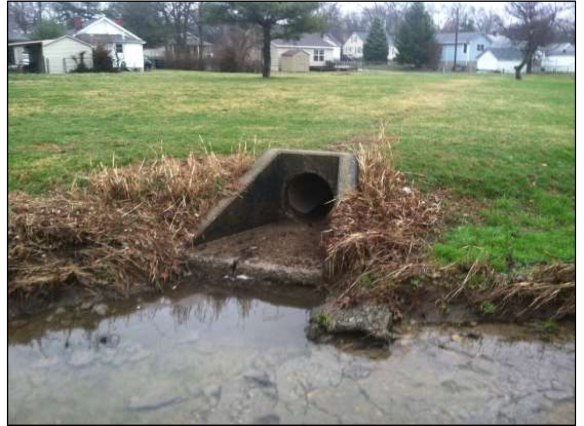
There were two stormwater outlets from adjacent neighborhood.
