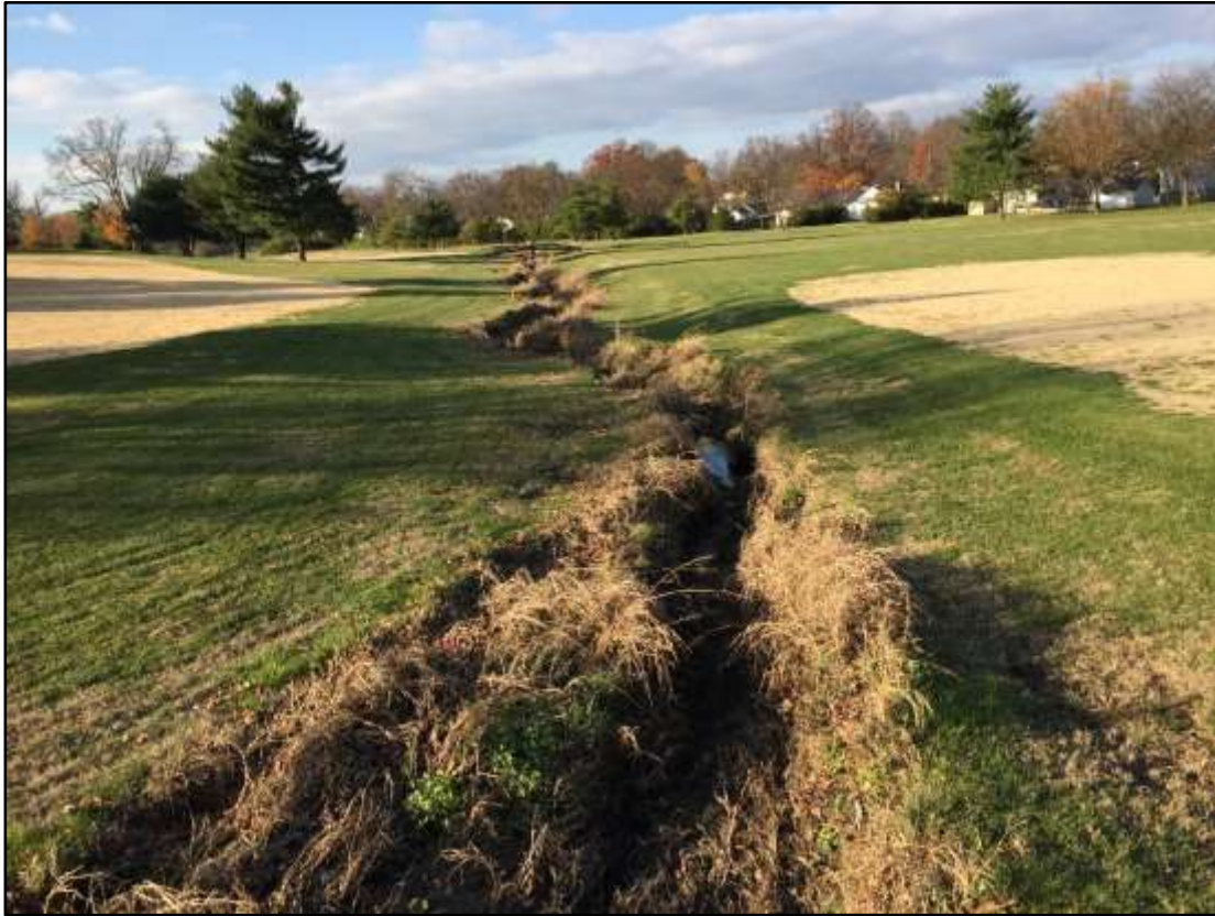
Lower reach was narrow and incised with eroding banks.
