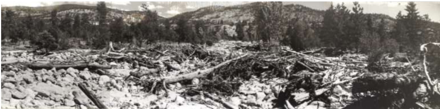
May 1942 – Flood damage from of breach of EC No. 4 Deposition of Cobbles, Boulders and LWD
